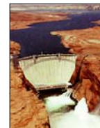
Glen Canyon Dam
